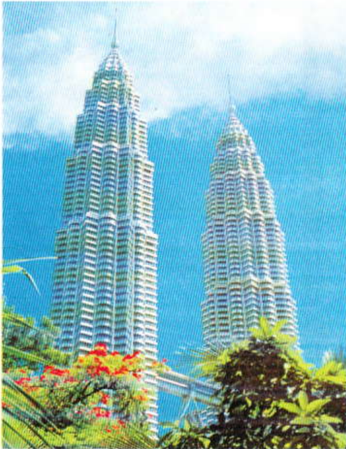
Petronas Twin Tower, K.L.
